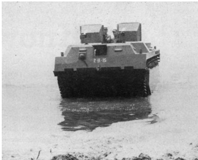
Two views of the LVT(3), which was the principal amtrac at Okinawa and into the postwar era.
