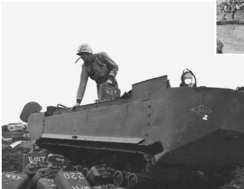
Iwo Jima 23 Feb 1945. First Combat appearance of the M29C "weasel" light amphibious vehicle—used for frontline resupply of high priority items. USMC Photo
