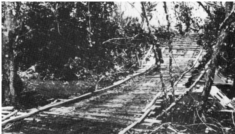
Amtracs used as pontoons over which wooden bridges have been built. Speed is of the essence during the initial landing hence the use of field expedients to span waterways.
